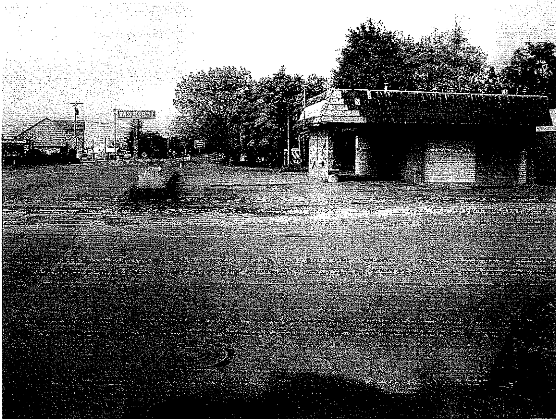
Photograph 9. Looking west toward Car Wash (former auto repair shop - 1920).
