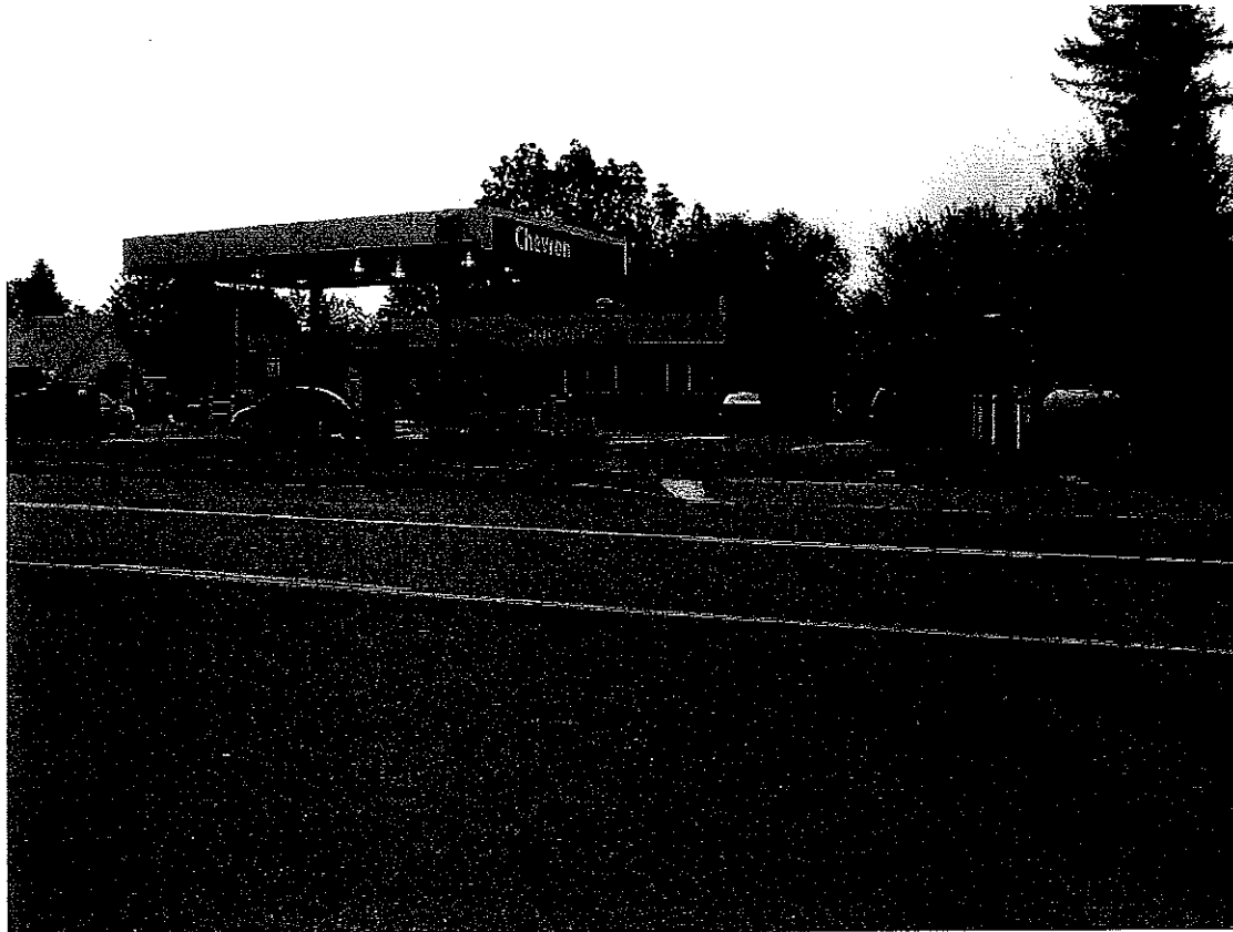
Photograph 6. Chevron station southwest of the intersection of OR228 and Washburn Street.
