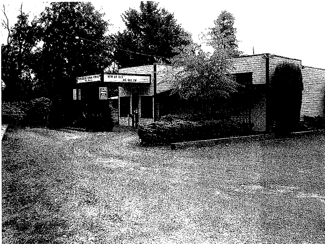
Photograph 16. Former truck repair shop adjacent to the south of OR228 at 221 Bishop Way.
